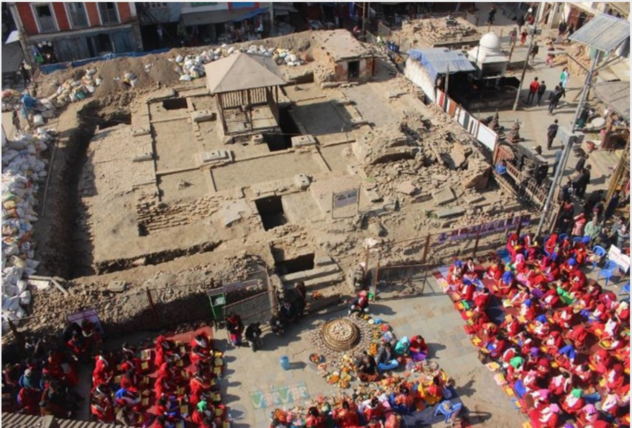
Post-earthquake rescue excavations at the Kasthamandap, Kathmandu, Nepal (Credit: Durham UNESCO Chair)
